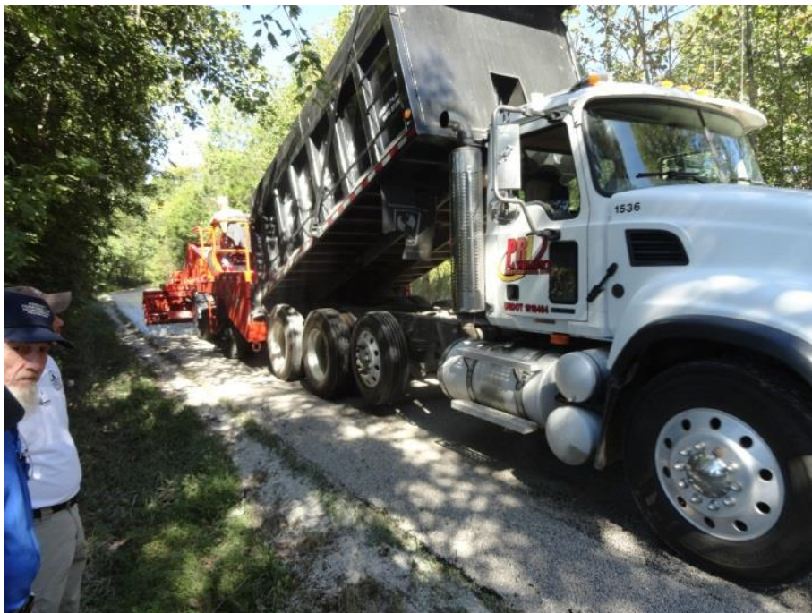
Rubber-modified asphalt chip seal application, Fleming County, KY. Photo by Christopher “Kitt” Tuttle
