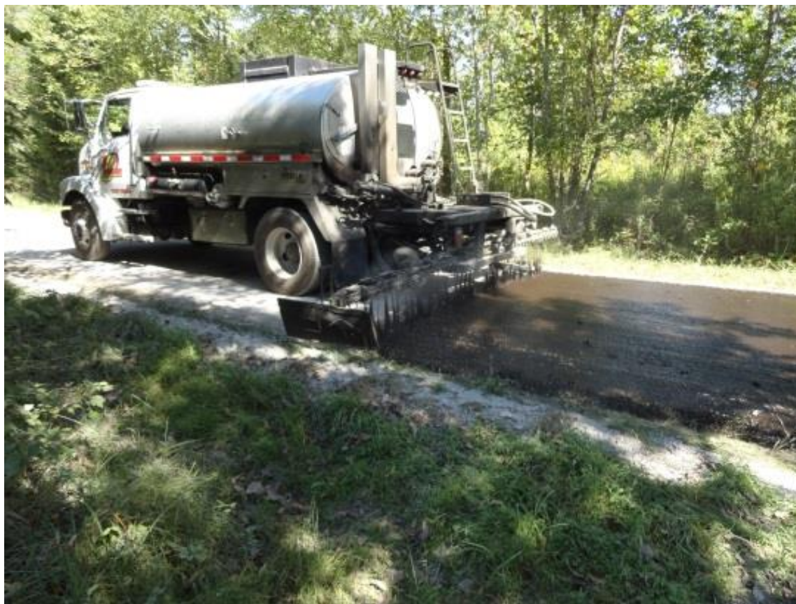
Rubber-modified asphalt chip seal application, Fleming, KY. Photo Christopher "Kitt" Tuttle
