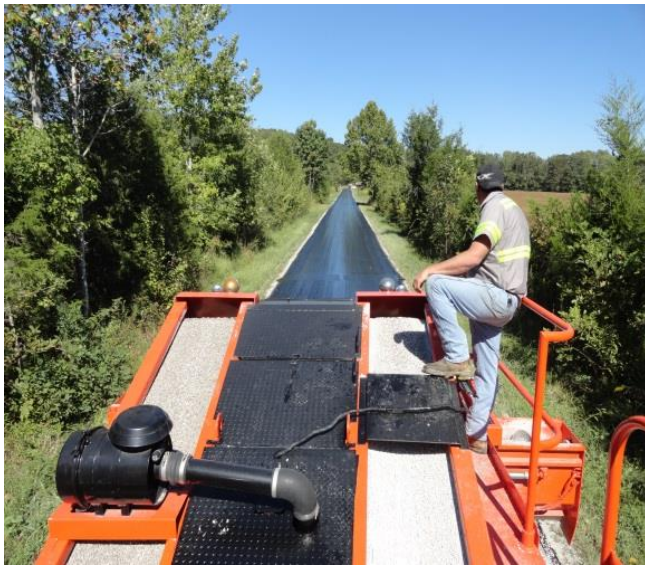
Rubber-modified asphalt chip seal application, Fleming County, KY. Photo by Christopher "Kitt" Tuttle
